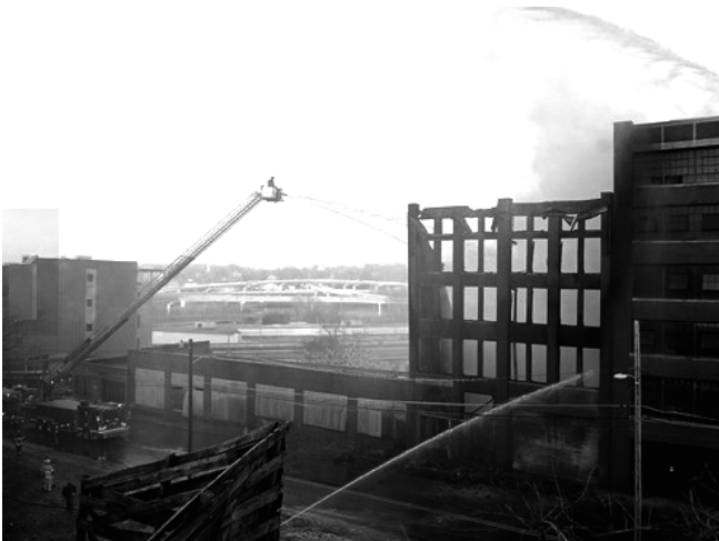
Figure 3. Jackson Avenue warehouse district fire: 2014
